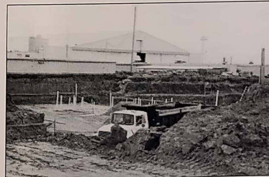
The dirt is piled high. The hole is dug deep. But when phase one is complete, the 513th ACG will have a new high-tech home to move into which will carry them into the next century.
